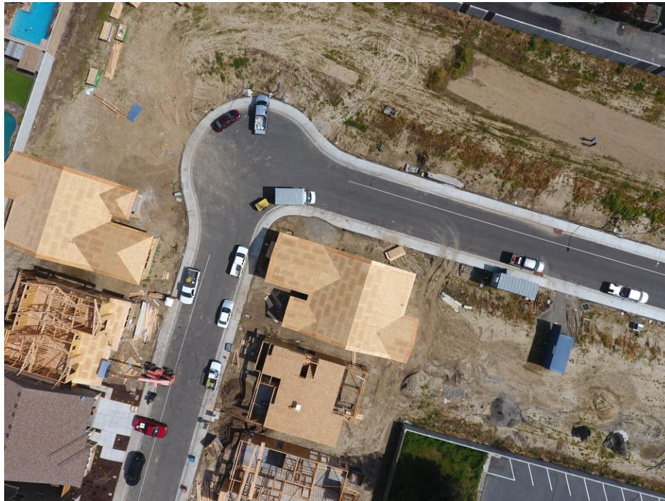
Neighbourhood construction. Source: Scott Blake on unsplash
